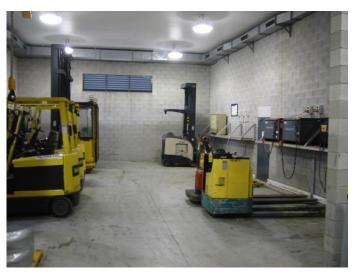
There have been a number of reported fire losses involving these units, principally during the recharging process. Insulation, battery boxes and accumulated grease deposits on battery powered trucks are combustible material which may become ignited and involve the truck in fire.
